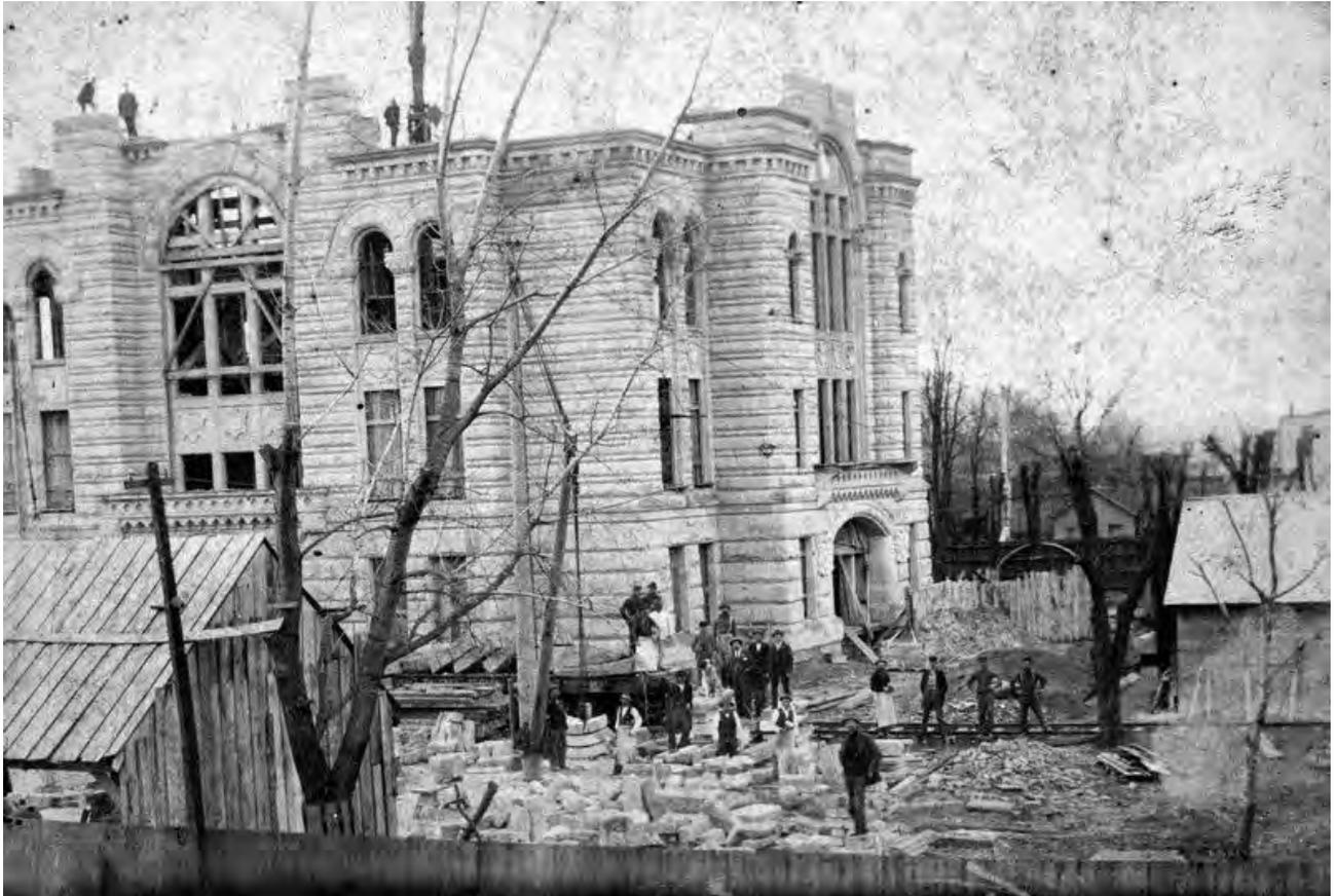
**The Knox courthouse was under construction from 1897-1898. A temporary railroad track was used to move heavy equipment and stone blocks. (Photo courtesy of the Starke County Historical Society)**
